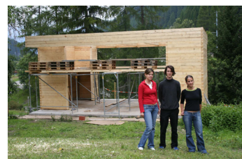
building process of the pavilion
