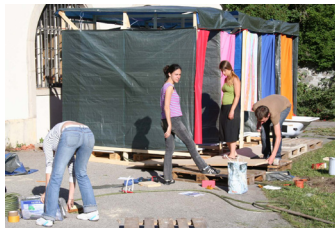
installation of the showers
